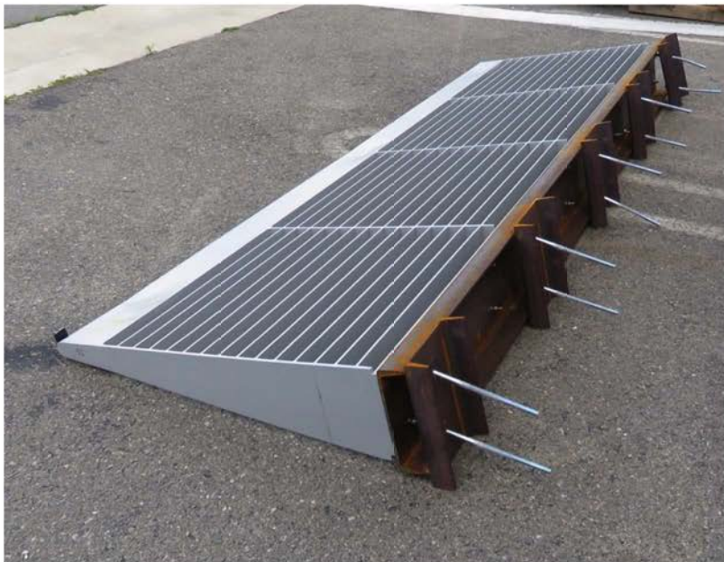
Can see 10" long 1/2" diameter bolts through back that went through the 6" x 12" wooden beam.
